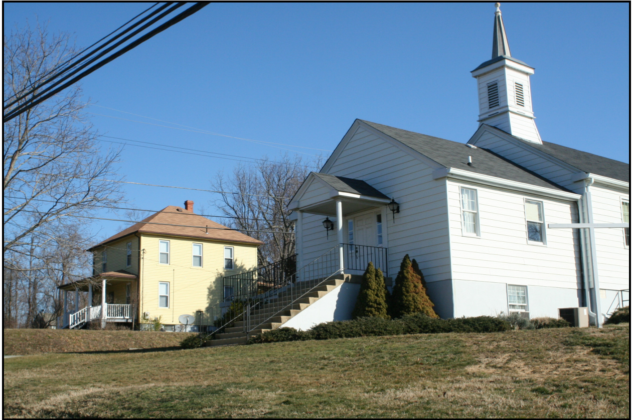
Looking northeast, Bowie Methodist Church, 8807- 8811 Maple Avenue ( EHT Traceries, 2008 )
