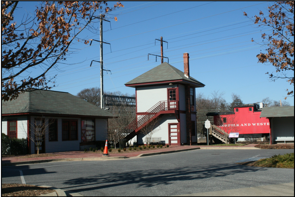
Looking northwest, Bowie Railroad Buildings (PG: 71B-002-09, NR), 8614 Chestnut Avenue ( EHT Traceries , 2008)
