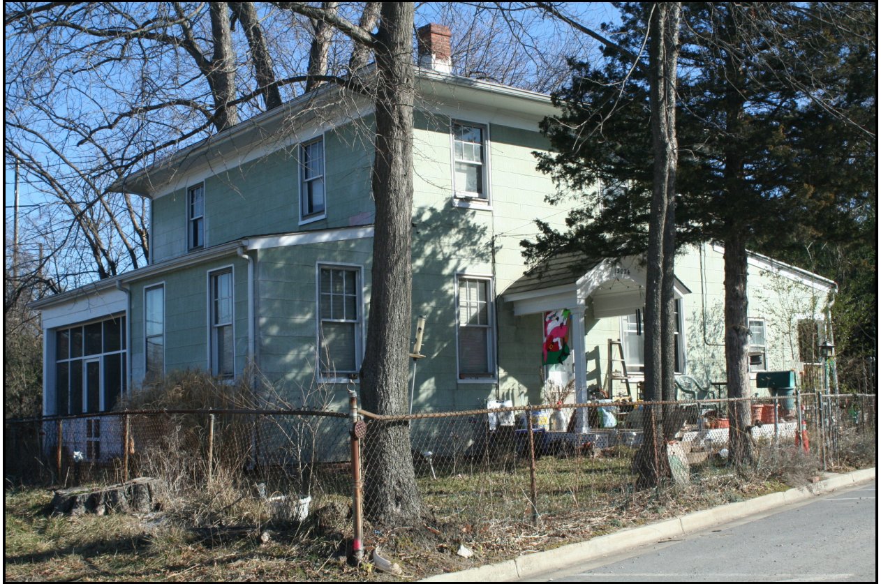
Looking northeast, 13024 11th Street ( EHT Tracerics, 2008 )
