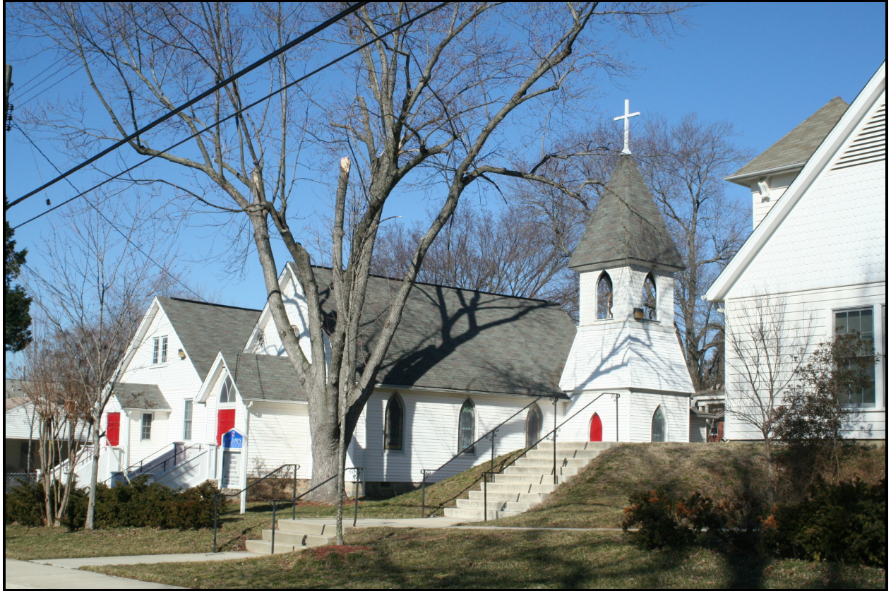
Looking northwest, St. James Episcopal Church (PG: 71B-002-05), 13010 8th Street ( EHT Traceries, 2008 )
