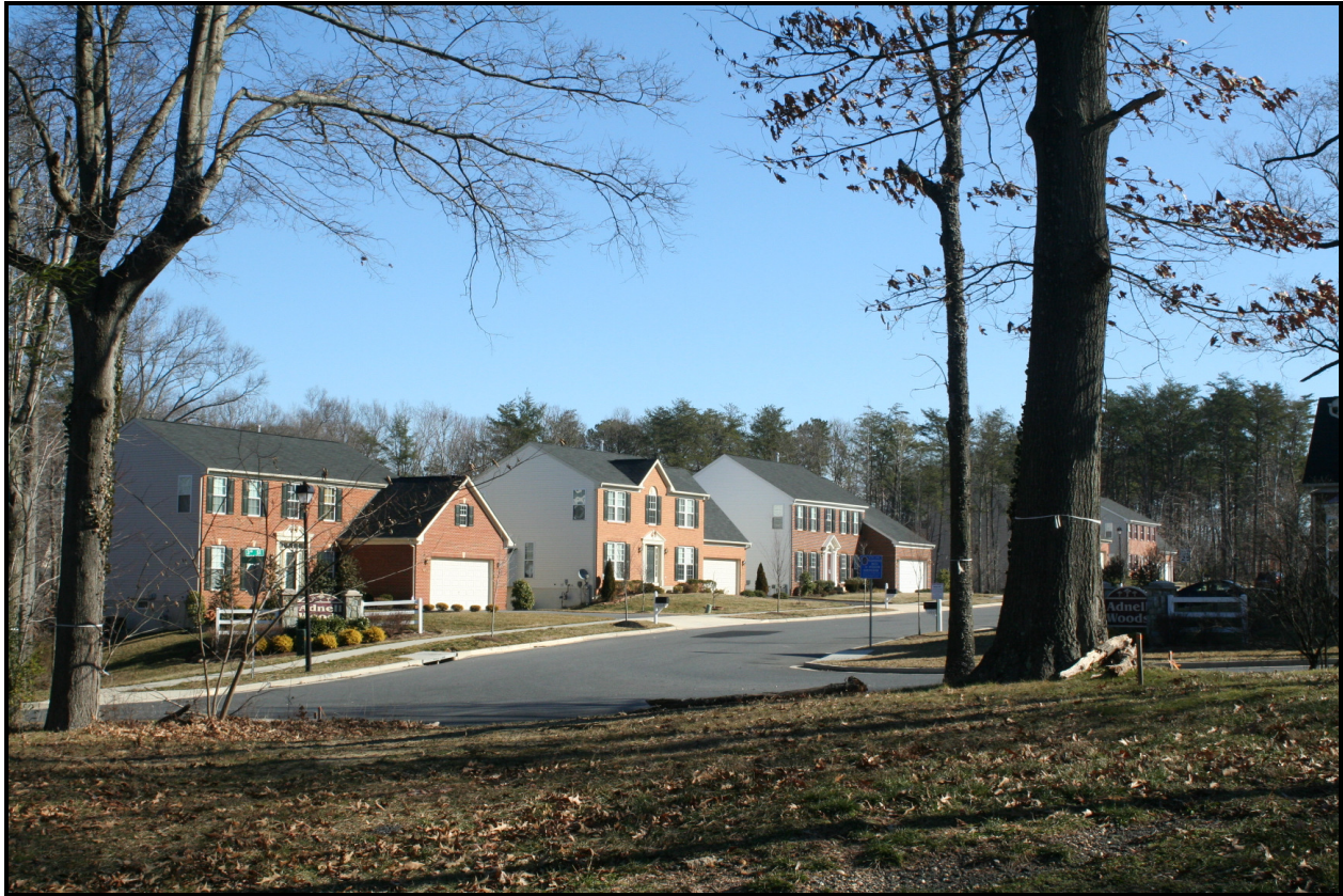
Looking northeast, 1300 block (even) of 3rd Street, Adnell Woods ( EHT Traceries , 2008)
