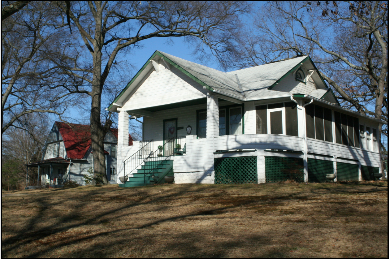
Looking northwest, 12906-12900 10th Street, William Luers House (PG: 71B-002-14) ( EHT Traceries, 2008 )
