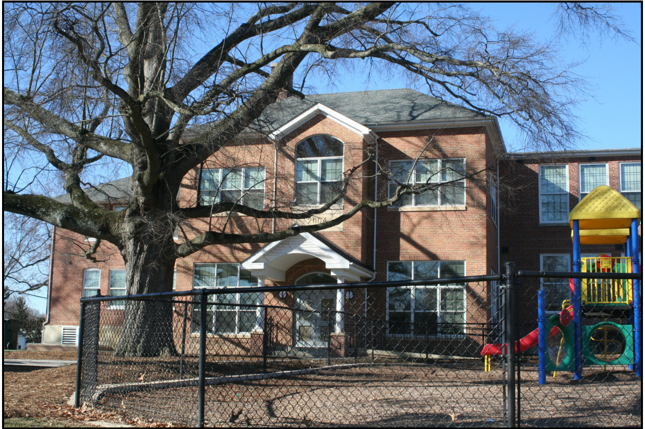
Looking northeast, Huntington Community Center, 13022 8th Street ( EHT Traceries , 2008)
